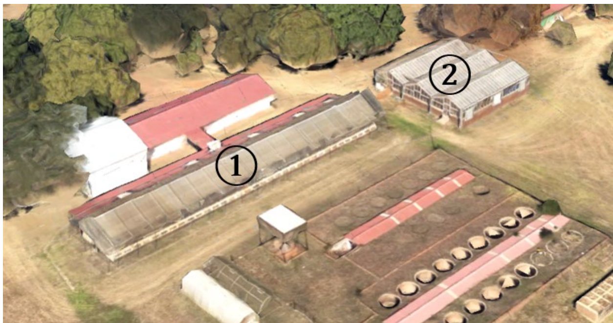
Figure 1: This project focuses on two steel-framed heritage greenhouses i.e. Greenhouse 1 and Greenhouse 2 (Davey & van der Merwe, 2023).
